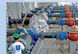
Stations de Pompage Pumping Stations
